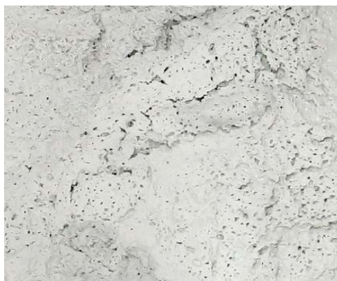
AFTER PARTIAL DRAINING
